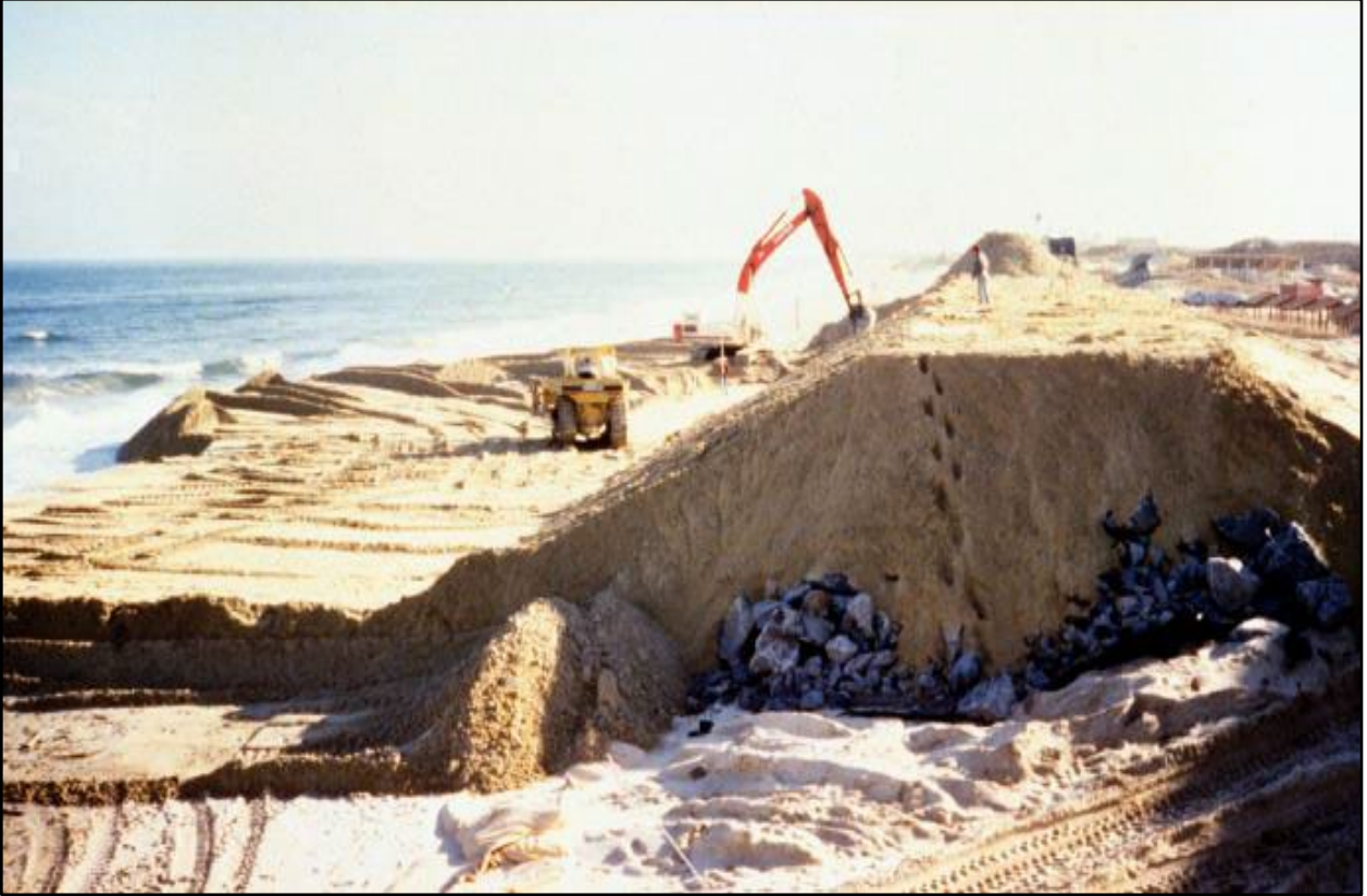
FIGURE 9.—Construction of a composite seawall in New Jersey. Illustration credit: USACE (2018a).
