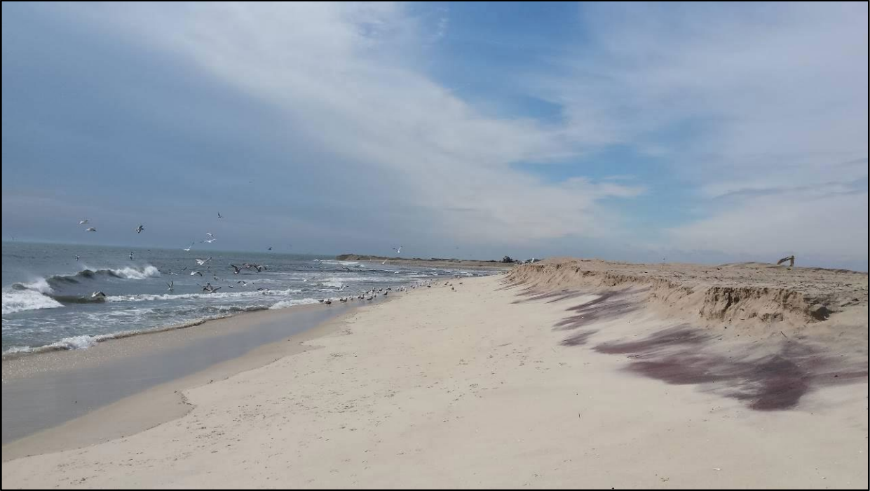
FIGURE 30 .—A widened berm and scarp formation at Smith Point County Park, Suffolk County, New York, during construction of the Corps’ Fire Island Inlet to Moriches Inlet Stabilization Project. Photo credit: Steve Papa, USFWS, March 2015.
