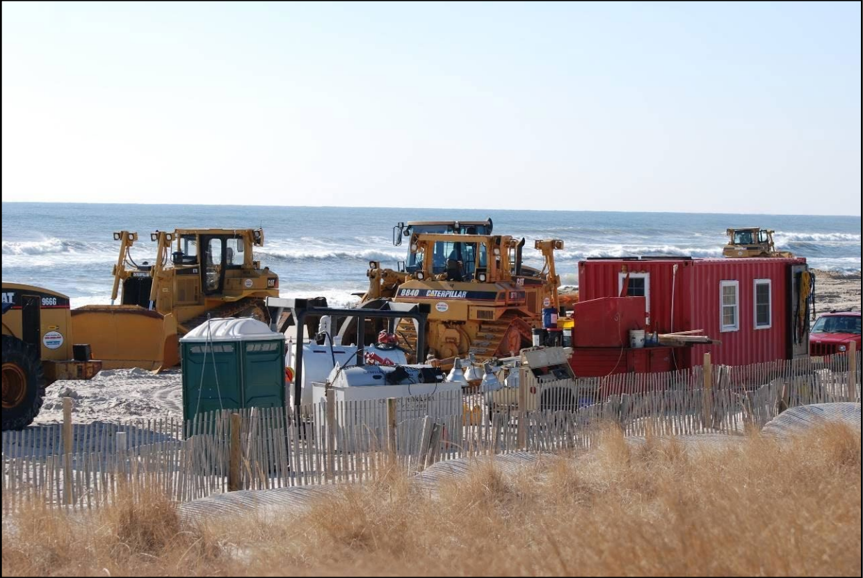
FIGURE 27.—Beach nourishment equipment on the beach. Photo credit: Steve Papa, USFWS, 2004.
