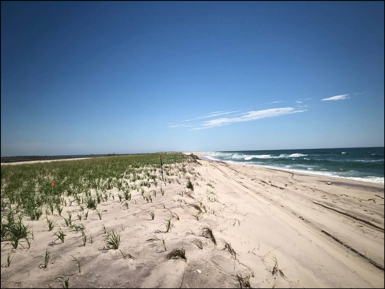
FIGURE 31 .—Erosion of nourished beach within the Corps’ FIMI Project area 3 years after construction. Narrowing of berm seen in foreground. Extreme erosion seen in shoreline at top of photo. Photo credit: Steve Papa, USFWS, 2018.
