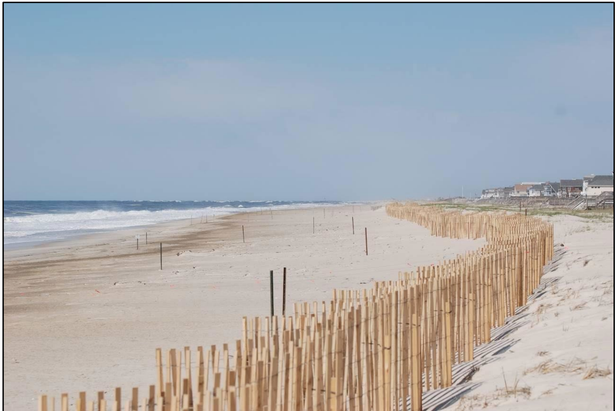
FIGURE 29.—Sand fence installed in the Corps' Westhampton Interim Storm Damage Protection Project area to promote lateral expansion of the dune at the expense of berm habitat. Photo credit: NYSDEC 2012.
